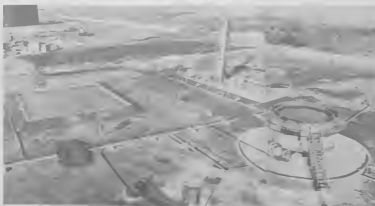
Partial view of improved fire training facilities. Vista parcial di facilidatnan mehora pa sinja paga candela.
